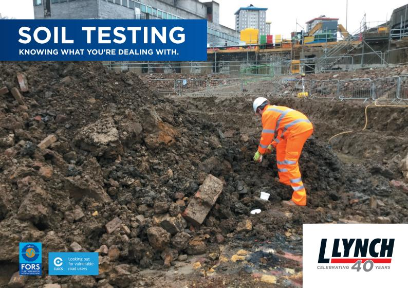
Before starting a construction project, the contractor must classify their waste leaving site, soil testing will identify contamination issues or to classify waste for disposal.
